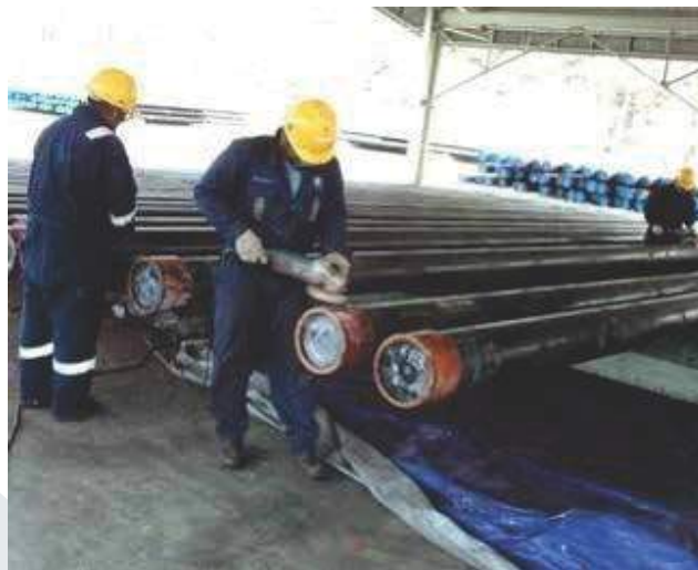
Cleaning of 9-5/8 Casing pipe for Inspection
