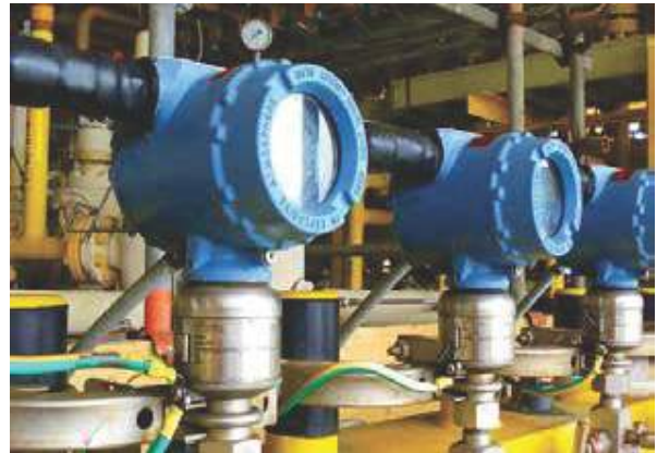
Replacement of instrument control system
