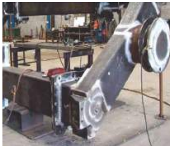
Finished MPI on offshore Structure
