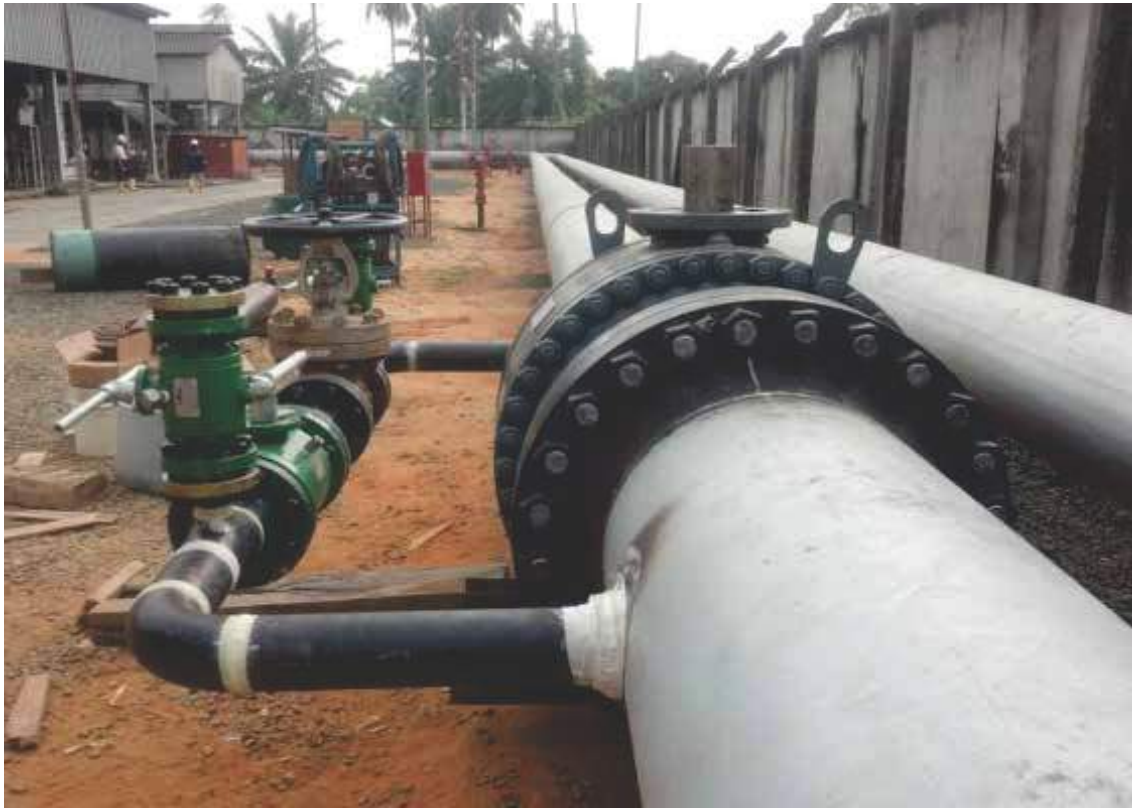
Installed Fabricated by-pass line
